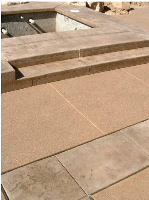
Light architectural exposed aggregate and stamped concrete are popular decorative finishes for penetrating sealers.
