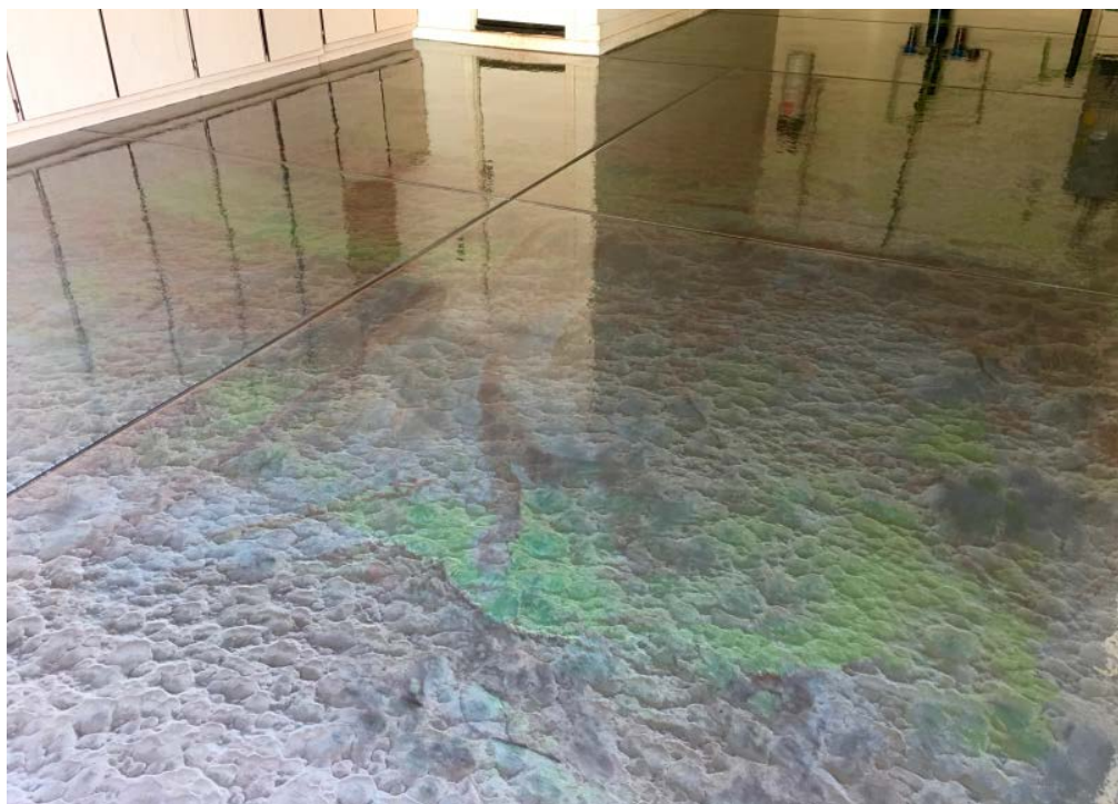
Photo courtesy of Jon Kopp/Quality Epoxy
