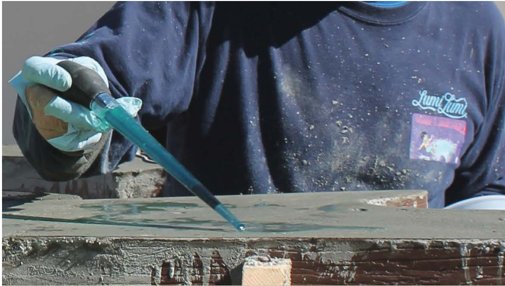
Much like an artist uses a brush for creative effects, Ralston sometimes uses a turkey baster filled with retarder to expose aggregate for stunning results (below).
