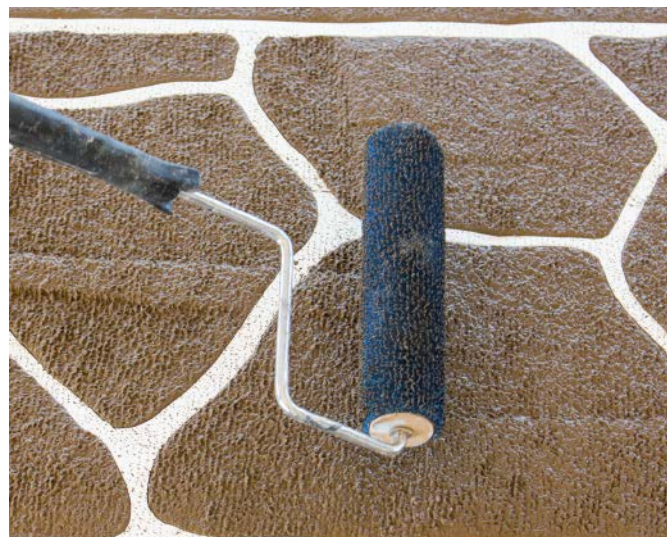
Rolling texture over a stencil can create the look of stone or brick in a fraction of the time it would take to build with the real thing.
