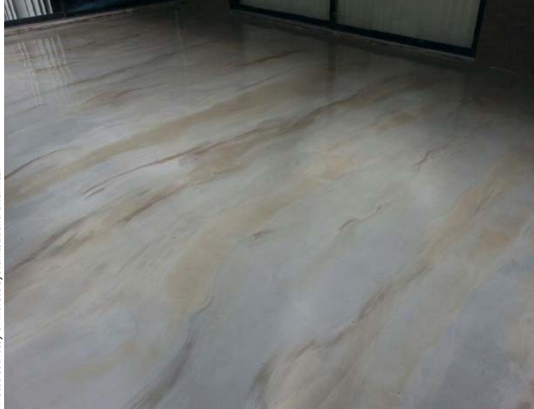
This Florida patio was created with Increte Systems' Level Top SP in a base color quickly followed by two integrally colored mixtures. The highlights were applied very quickly and hit once with a magic trowel/squeegee to achieve this polished marble-like surface. After curing, the patio was sealed with Increte's water-based urethane. Work was done by Matt Johnson with Mr. Epoxy and Paint in Sarasota.
