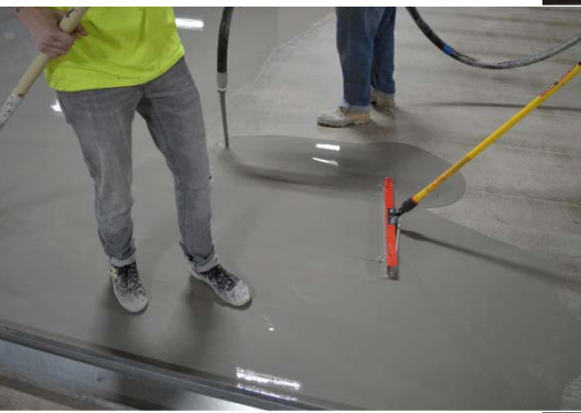
Ardex K 10 — a reactivatable, high-flow, self-leveling underlayment — was used on the floor of this high-technology manufacturing facility in Utica, New York.
