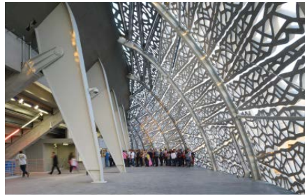
The Stade Jean Bouin in Paris, France Photos courtesy of American Concrete Institute
