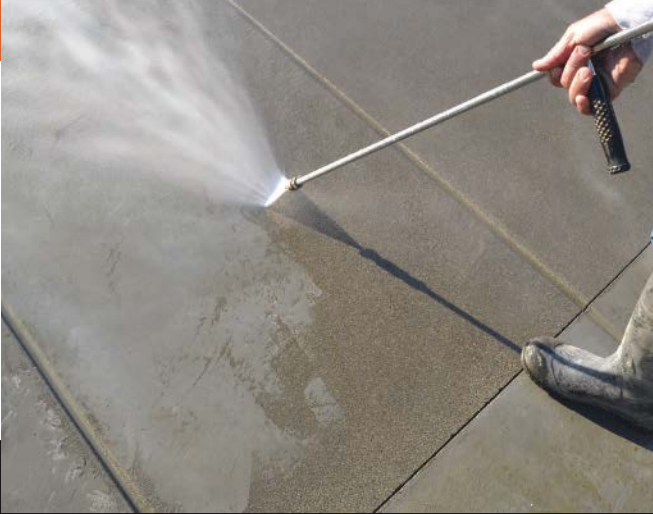
LITHOCAST Surface Retarders are available in six formulations ranging from light to heavy aggregate exposure
