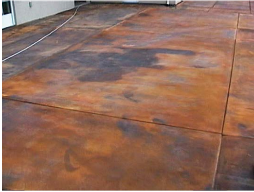
High loadings of fly ash or chloride accelerator can create blotchy and inconsistent effects when staining.
