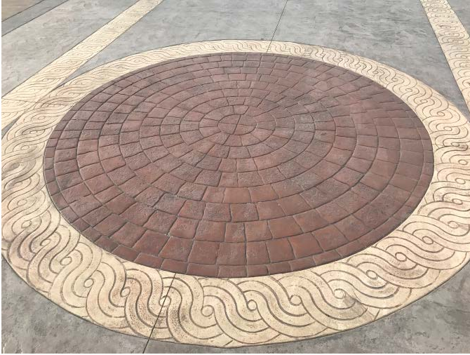
Cast-In-Place Stamped, Over 5,000 Square Feet, First Place Bomanite of Southeast Asia, Quezon City, Philippines Oasiz Hotel
