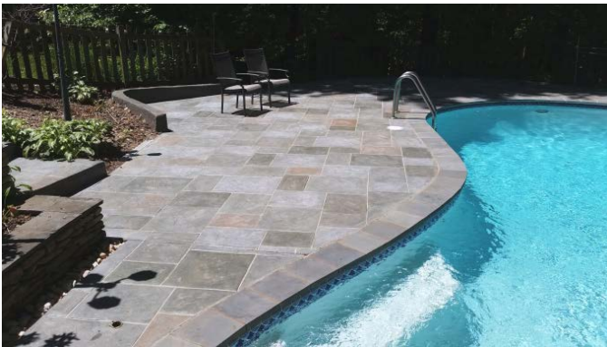
Cast-In-Place Stamped, Under 5,000 Square Feet, First Place Salzano Custom Concrete, Centreville, Virginia Faux Bluestone in Overton
