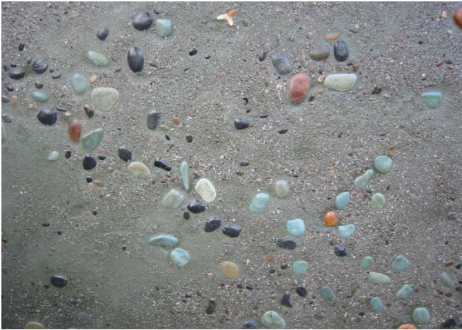
A closeup of sunburst cobble reveals several colors including jade green, Kuro black and Five Springs. This installation, at a coffee café entrance, features aggregate bands in areas of green-colored concrete, conveying a marine motif.
