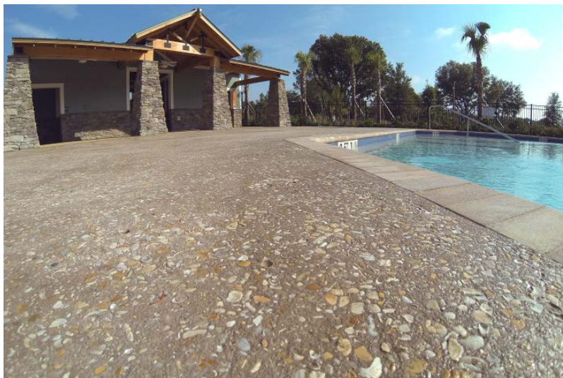
This gray-concrete pool deck was blasted to take the edges off the shell aggregate. Integral coloring was used in the miniature golf project.
