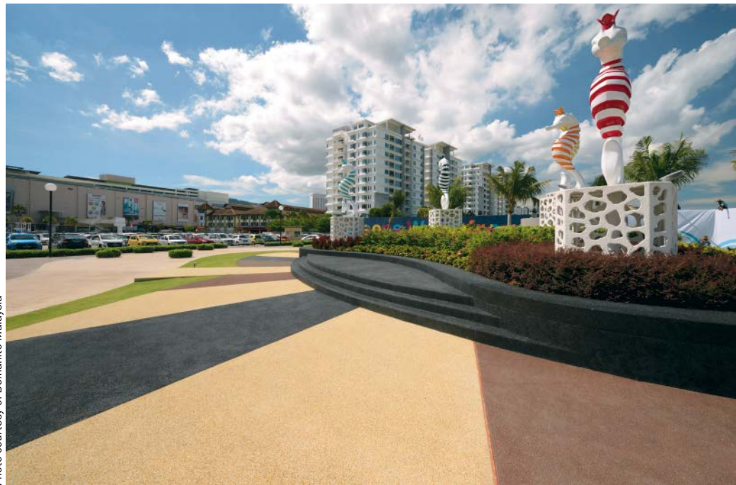
Integrally colored exposed aggregate and textured concrete deck out the entrance of the Queensbay development in Penang, Malaysia.
