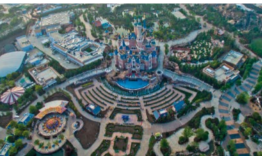
More than 1 million square feet of decorative concrete was installed at the Shanghai Disney Resort that opened in 2016 in Pudong, Shanghai, China.
