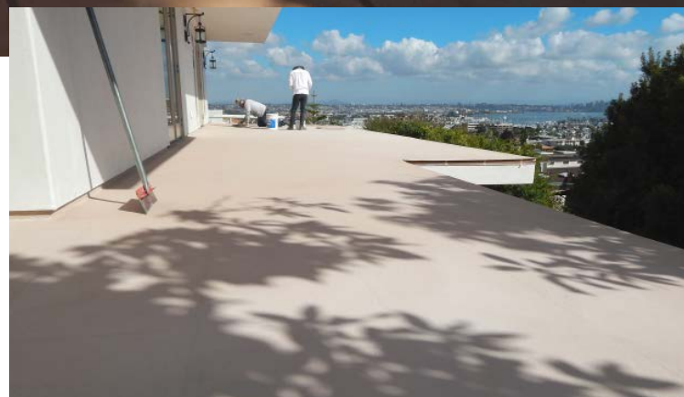
Seen here is a wooden deck in Point Loma, California, before and after Kaimana Coatings installed a decorative waterproofing system over it.
