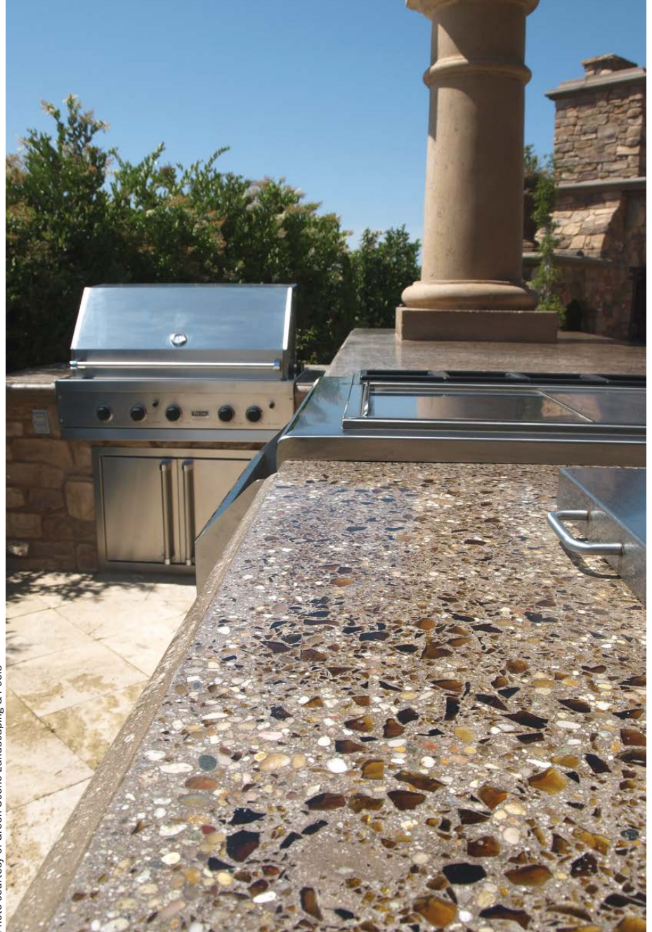
Seen here is a Green Scene Landscaping & Pools polished countertop with beer bottle glass aggregate. Company owner Scott Cohen says he prefers IPAs but any glass will do.
