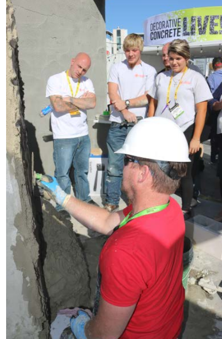
Photos by Concrete Decor staff
