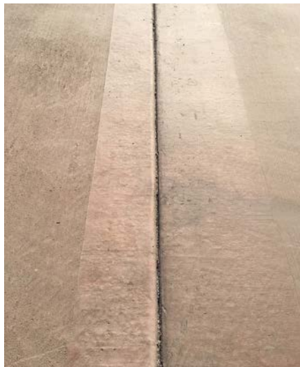
Care should be taken to ensure that the same size edger groover is used to avoid making costly mistakes in aesthetics.
