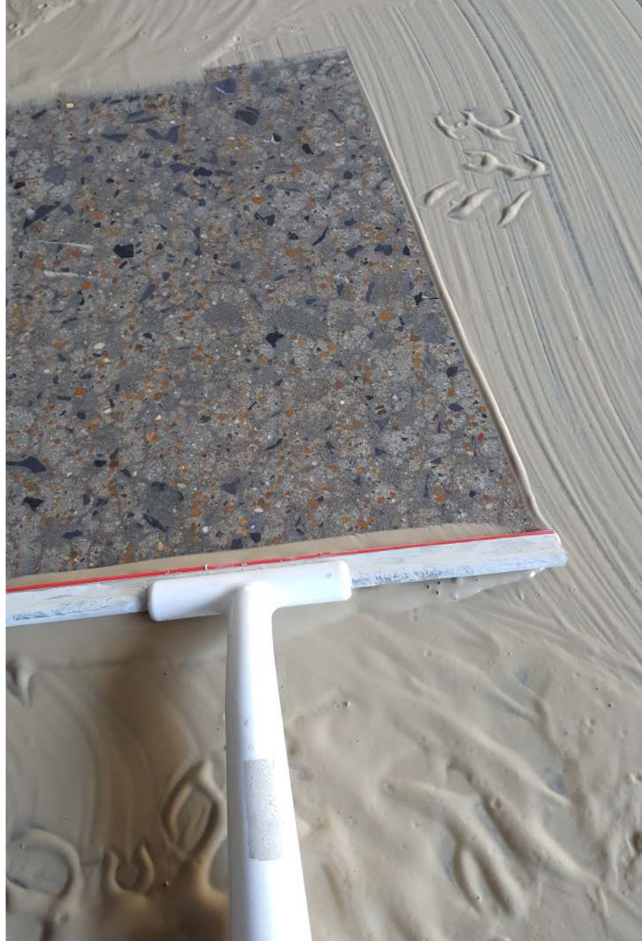
A squeegee pulls the KickStart slurry away from the floor so the installer can evaluate how well the large aggregate has been exposed.
