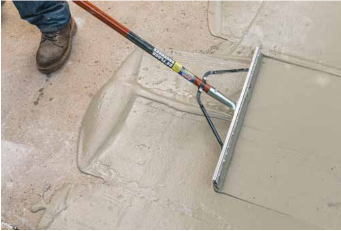
Resurfacers are applied to concrete surfaces in very thin layers. They are great products to use when it comes to repairing cracks and chips.
