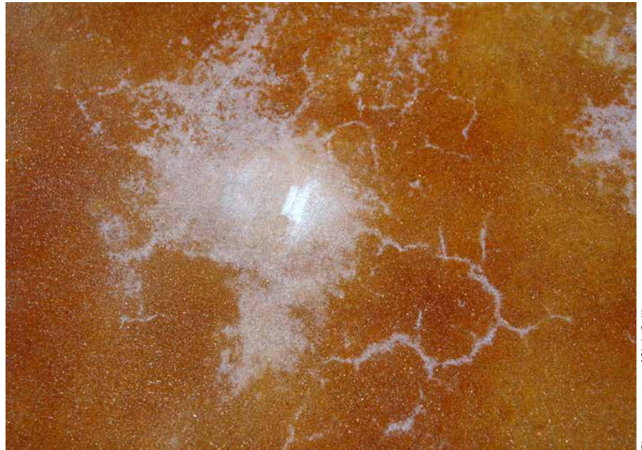
This sealer failure was caused by condensed moisture in a low spot on the floor that created an area that fell below the minimum film-forming temperature.
