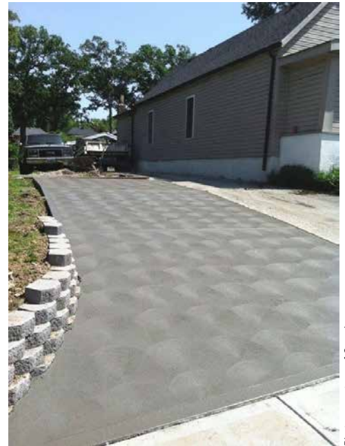
Gray concrete finished with a half-fan technique can be impressive.
