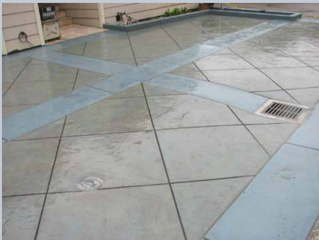
Parallel and perpendicular colored bands interface with diagonal deep joints in the panels.
