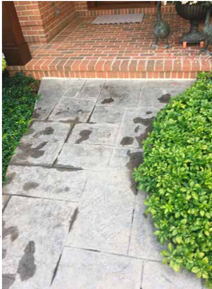
This stamped concrete walkway's original color was extensively faded but was transformed beginning with a thorough scrub and power wash. This was followed by an application of a light charcoal concrete stain and two coats of a sealer with a satin finish.
