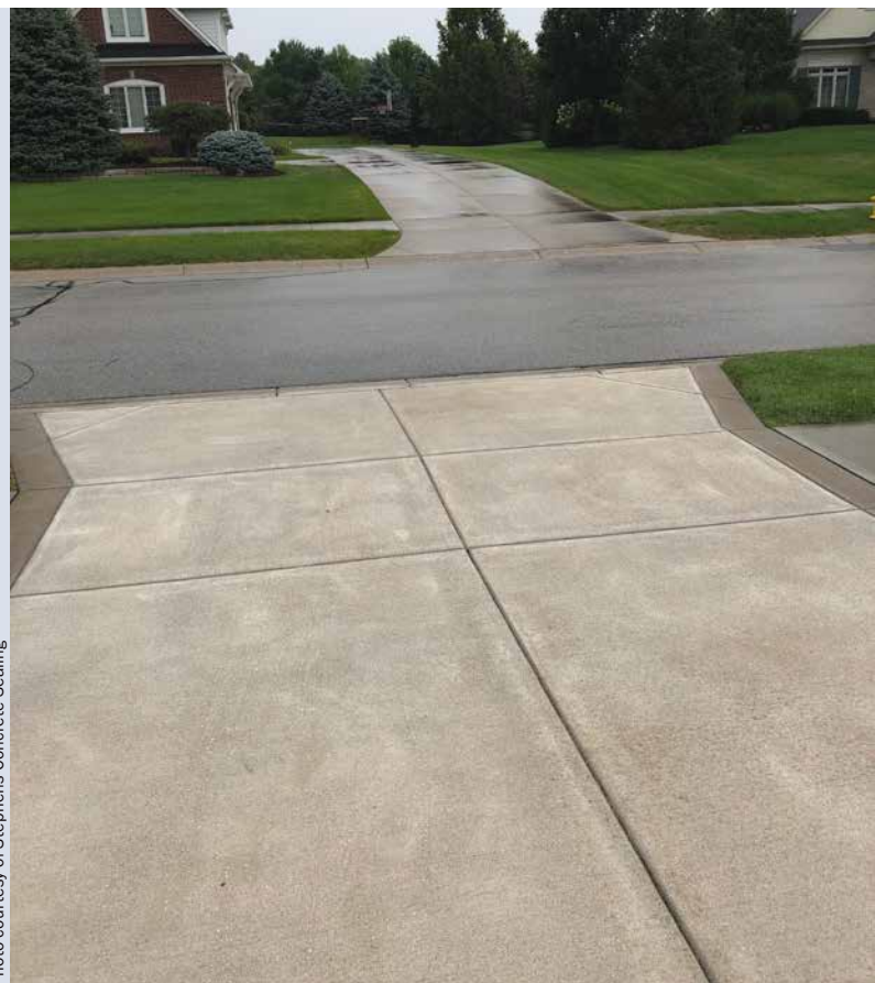
Photo courtesy of Stephens Concrete Sealing
