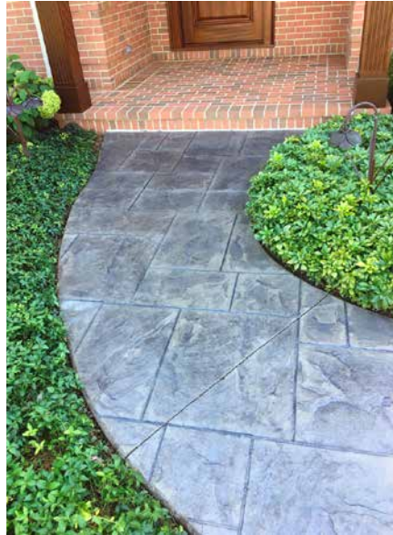
This stamped concrete walkway's original color was extensively faded but was transformed beginning with a thorough scrub and power wash. This was followed by an application of a light charcoal concrete stain and two coats of a sealer with a satin finish.
