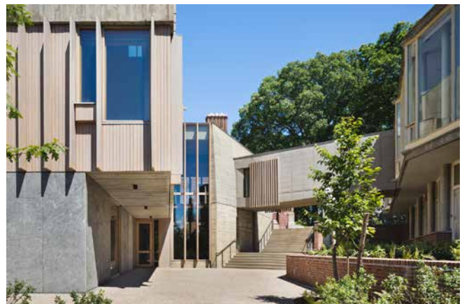
Vertical/Facades, Over 5,000 Square Feet, First Place Consigli Construction Co., Milford, Massachusetts Wellesley College Pendleton Hall West Addition
