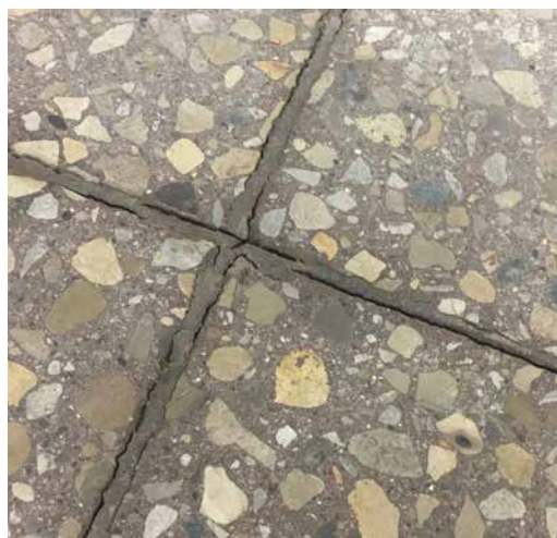
An aliphatic joint filler (left) won't split, pull away or discolor like an aromatic joint sealer (right) will.
