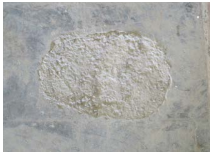
Trapped water-related delaminations come in all shapes and sizes. They can be roundish ( left ) in one spot and long and rectangular ( right ) in adjacent areas.
