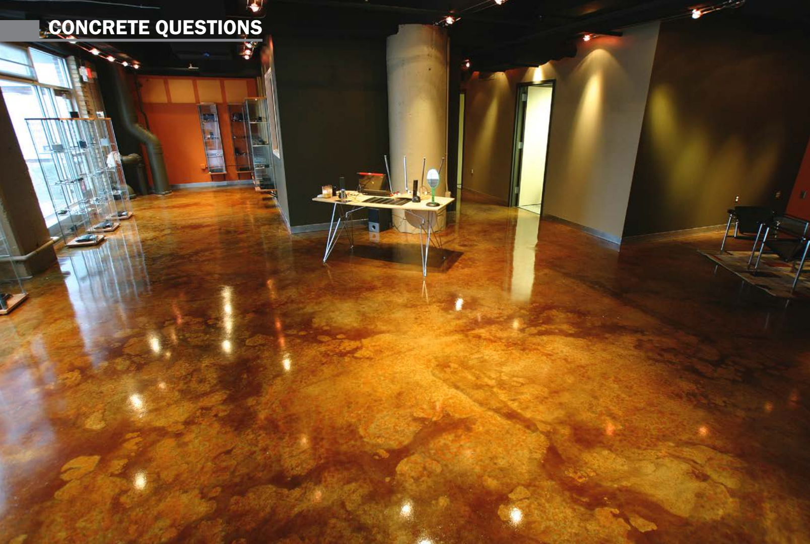
After allowing concrete to properly dry and cure, a surface can be stained and sealed with stunning results.
