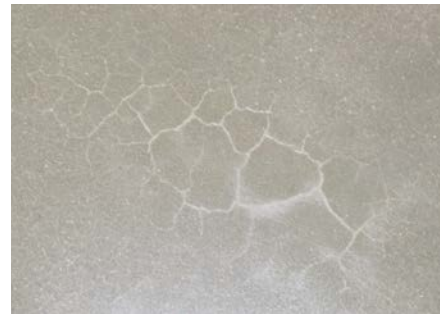
Trapped water-related delaminations come in all shapes and sizes. They can be roundish ( left ) in one spot and long and rectangular ( right ) in adjacent areas.
