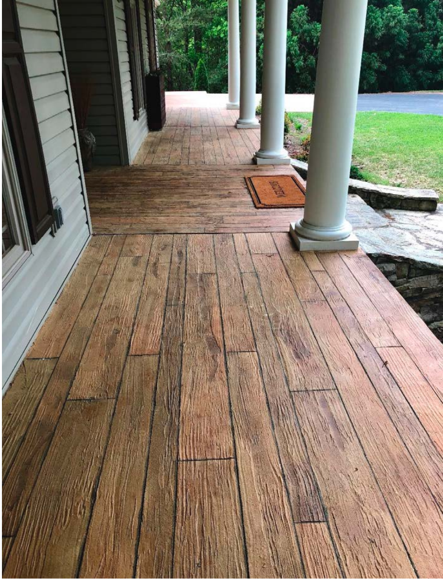
This front porch had a concrete surface to begin with and was rejuvenated with an overlay colored and sculpted to look like wood planks.
