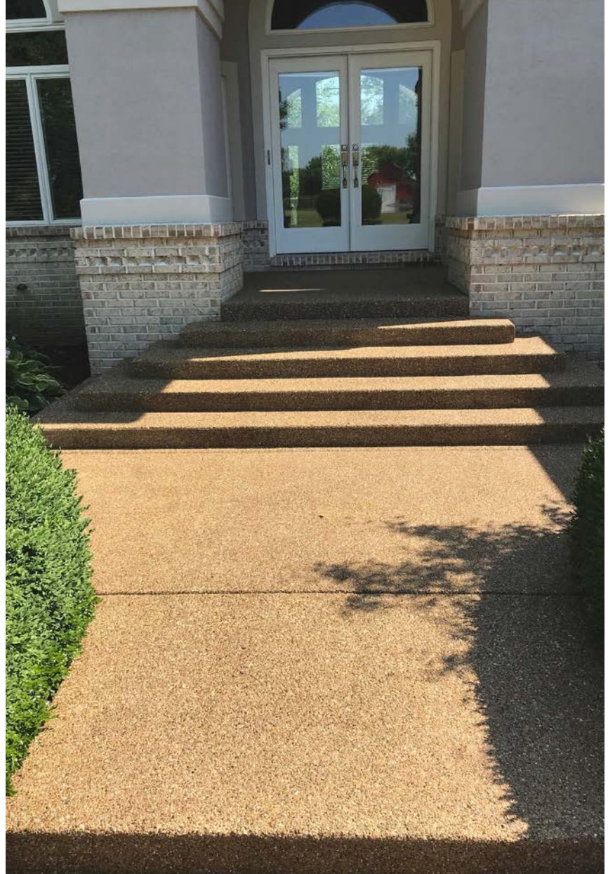
Eight out of 10 of Stephens Concrete Sealing's customers choose a honey brown-tinted high-gloss sealer for their exposed aggregate surfaces.
