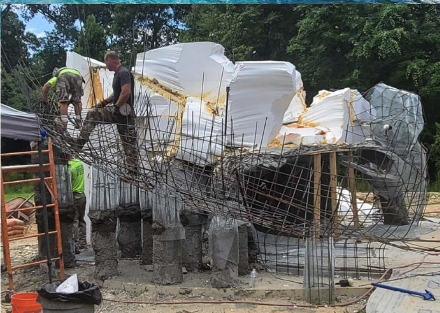
Photos courtesy of Beyond Vertical Concrete
