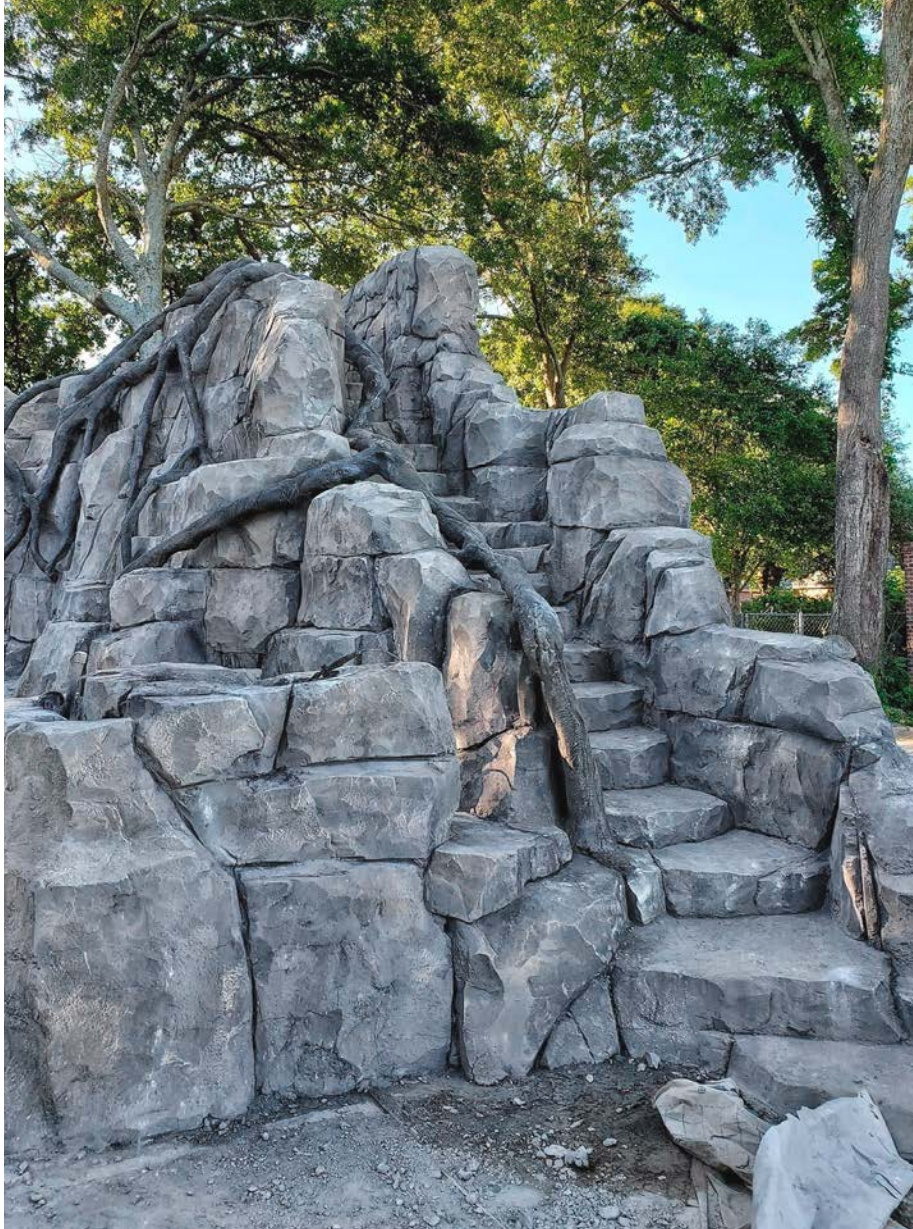
This foam-core construction staircase and fire bowl was built as part of a residential backyard project in Lafayette, Louisiana, done by Bask Pools and Beyond Vertical Concrete. It features 24 hand-carved steps leading to a 39-foot waterslide.
