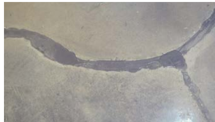
The only way to guarantee that a joint is completely filled is to slightly overfill it. When it's shaved, some residue will be left behind which a grinder will easily take off during the polishing process.
