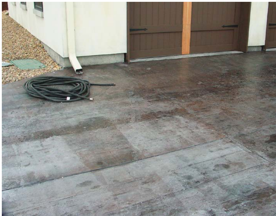
Applying a sealer that's high in acetone to a dark driveway in hot conditions may lead to rapid drying and blistering, and result in a blotchy and inconsistent finish.
