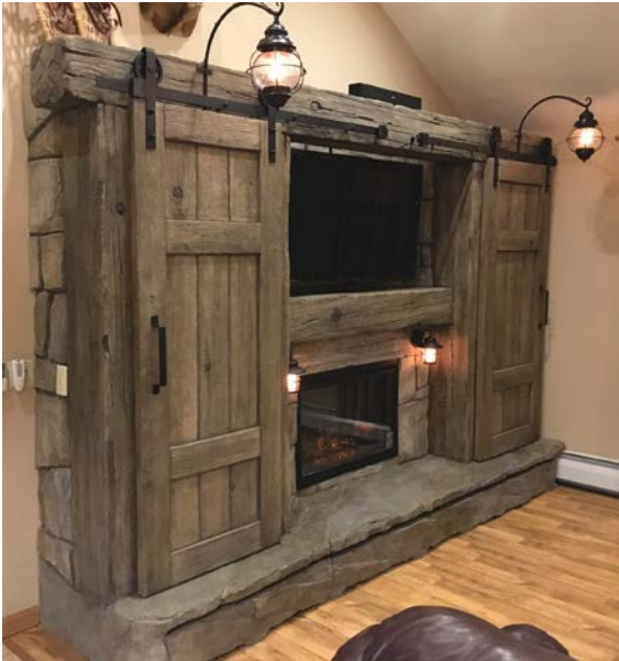
Vertical concrete isn't just being used to replicate a wide variety of stone. This handsome entertainment center may look like reclaimed barn wood, but it's carved concrete. The unit's operable doors are designed to slide back and forth.
