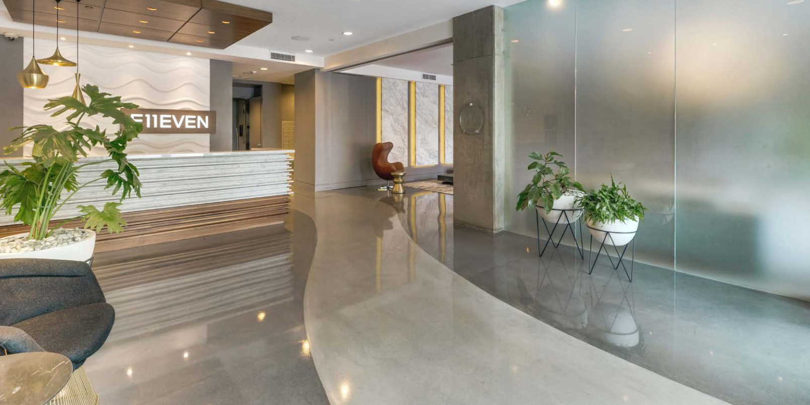
Although overlays are not new to the industry, the products today are much more long-lasting and harder than those offered in the past. GSPEC, a self-leveling product used to breathe new life into the lobby of this residential high-rise in downtown Los Angeles, is as durable as terrazzo without the busy aggregate-look. Photo courtesy of Green Chemistry Innovations
