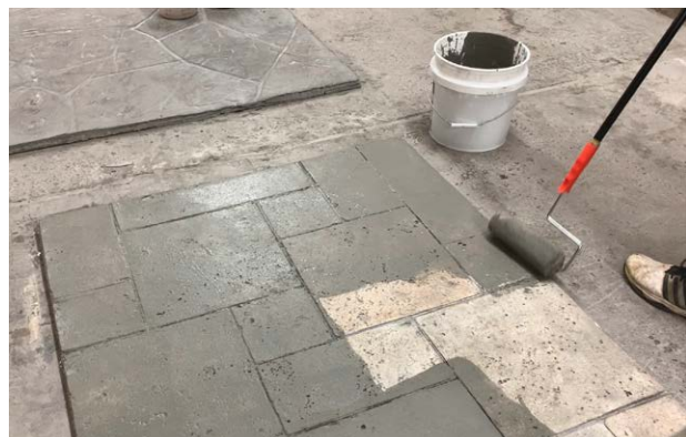
Some overlays can be rolled on a textured surface to take the color back to gray or white while leaving the texture.
