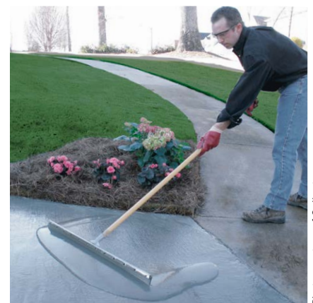
Installing an overlay is an affordable alternative to tearing out old and worn concrete driveways, sidewalks and patios and replacing them.
