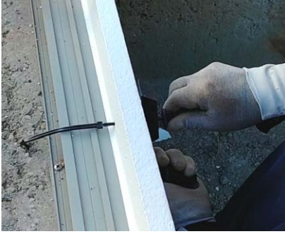
(Above) Mortex's Spear and Button anchoring system is one of the company's solutions to eliminate tie wires. (Middle and right) The company's reusable brackets in its Bracketit line are designed to adhere forms to various materials.
