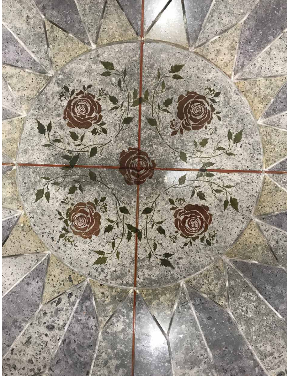
The roses and greenery in the center of the saw-cut showroom floor are made with Flattoo stencils from Surface Gel Tek. Stencils only comprise about 10% of the floor's design.
