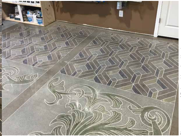
The office (left) and warehouse floors (above and far right) feature Venetian-inspired 3-D designs. All designs were cut free-hand with a 4-inch grinder.
