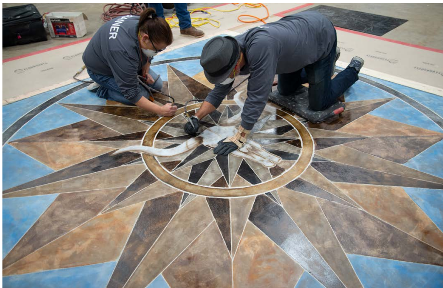
Debbie Ohland and Rick Lobdell used Engrave-A-Krete tools and SurfKcoat dyes to bring this engraving to life.
