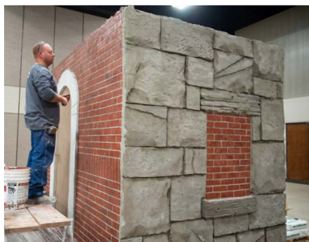
Photos by Concrete Decor staff
