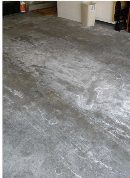
Polished concrete can experience efflorescence from moisture which looks like a whitish powder. The side effect is temporary.
