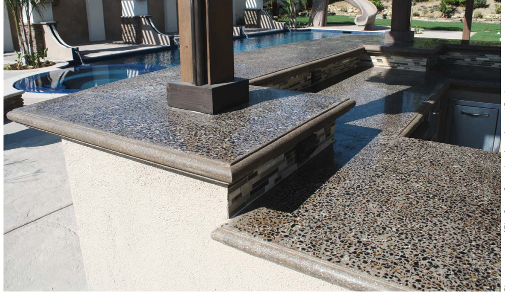
Combining materials — such as glass, colored aggregates, wood and metal in or around concrete — is a current micro-trend for cast-in-place concrete.
