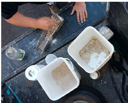
To make authentic-looking tabby, mix three parts white sand to one part white cement and cover the applied mortar with tiny shells and broken bits.
