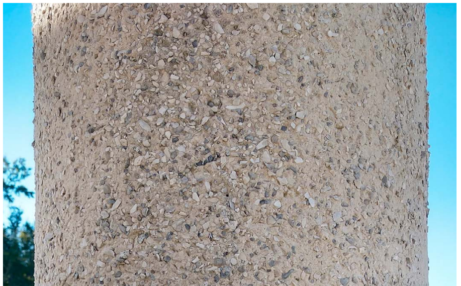
To make authentic-looking tabby, mix three parts white sand to one part white cement and cover the applied mortar with tiny shells and broken bits.
