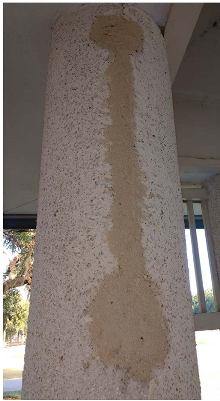
This left an area that needed to be patched with tabby.
