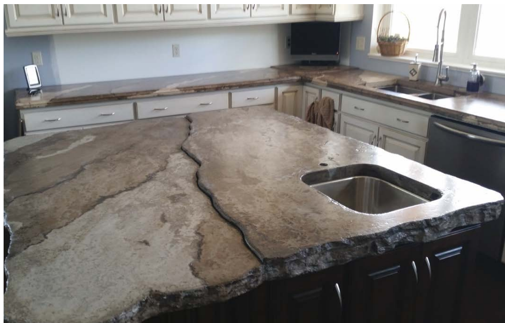
This bilevel top is formed with two pieces joined at a seam about midway.
