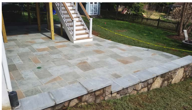
Photo courtesy of Salzano Custom Concrete
